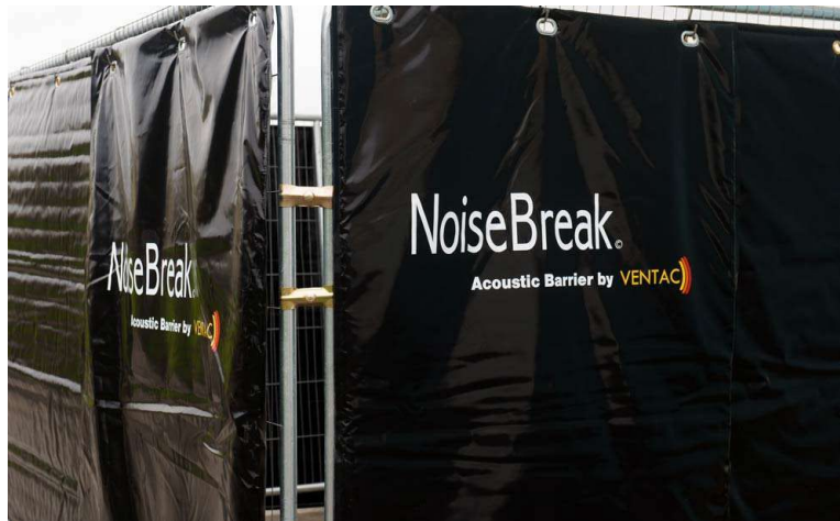
Chapter 10 Figure 10-1 Temporary Construction Noise Barrier © Ventac
